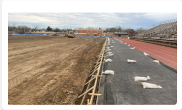
Ground Being Prepped
