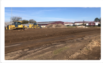
Grass Removed and Soil Readied
